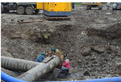
Study visit to gas pipeline rehabilitation site
